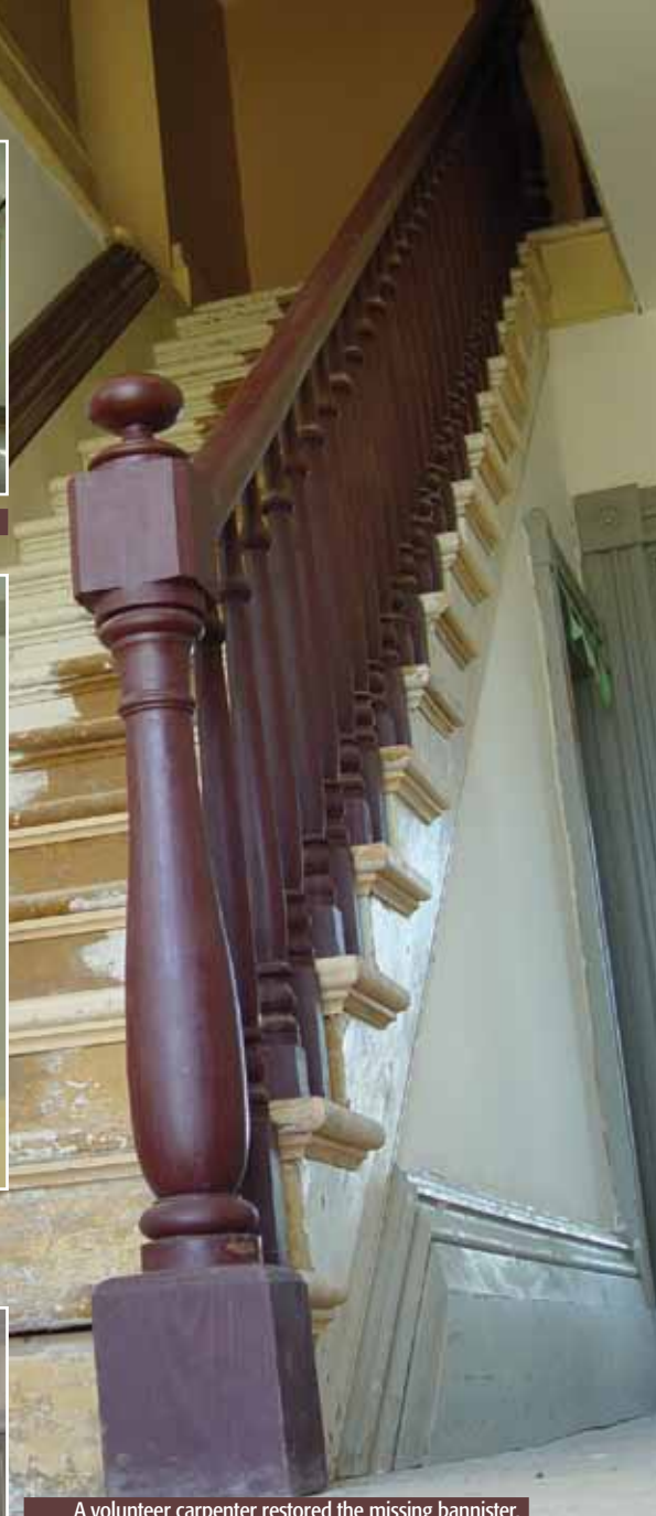
A volunteer carpenter restored the missing bannister.
